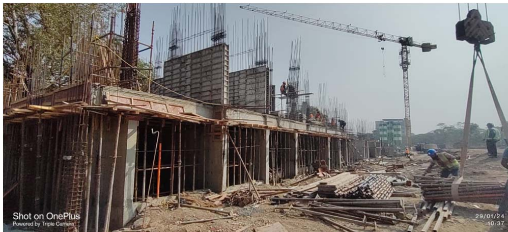
Wing D - Upper Gr. Floor slab completed
