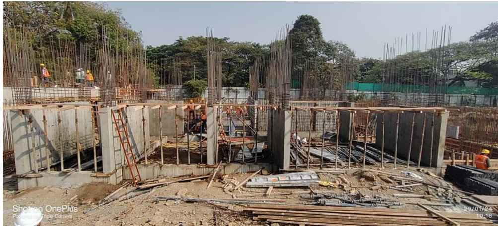
Wing E - Upper Ground Floor slab Work is in progress
