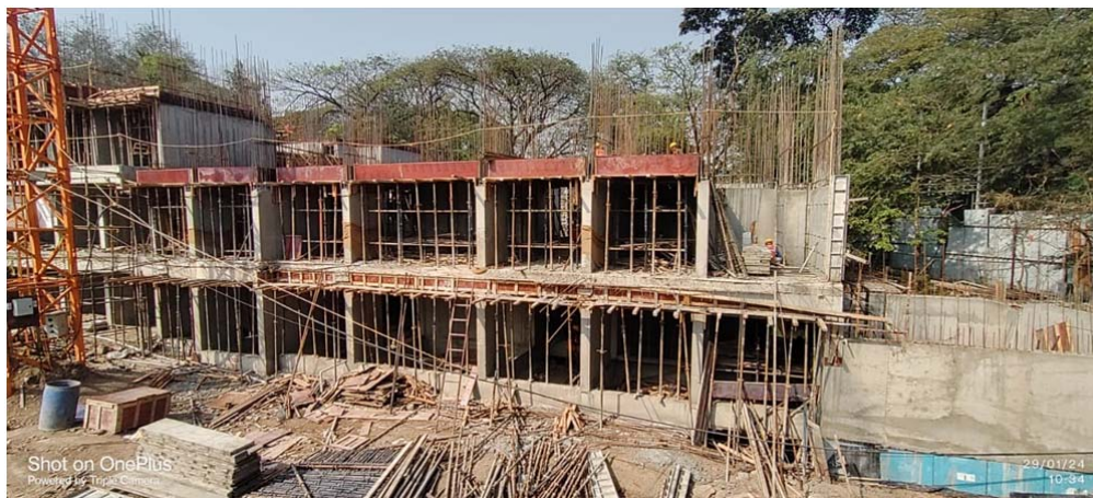
Wing C - Podium floor slab is in progress
