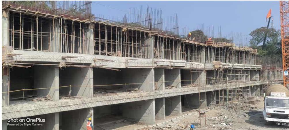
WING AB - 1 st Floor Slab is in progress
