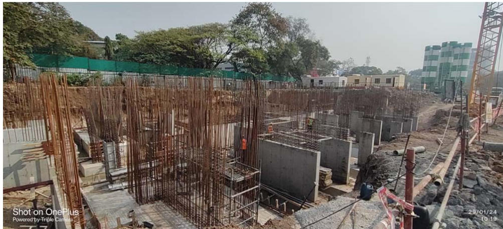
Wing F - Footing and Stub Column work in progress
